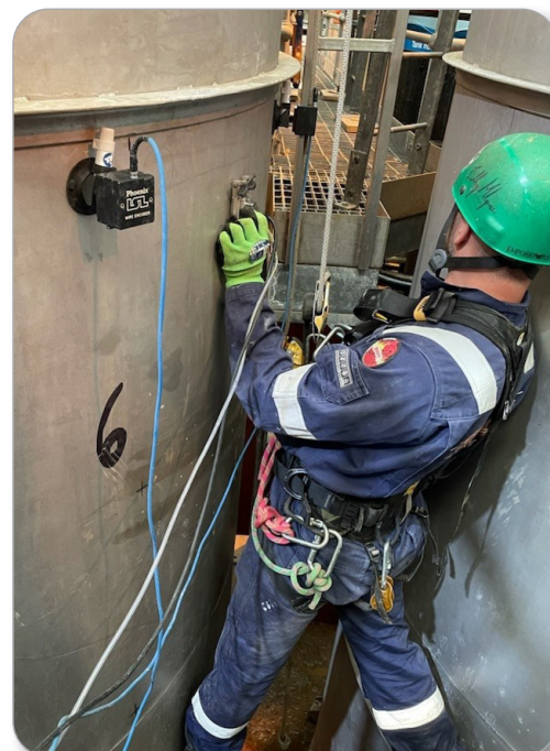
Corrosion Mapping on stainless steel tank
